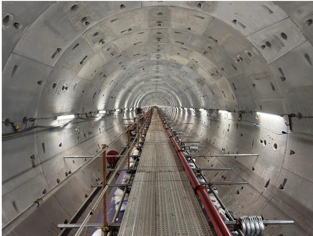
Interior of 6m diameter subsea tunnel
